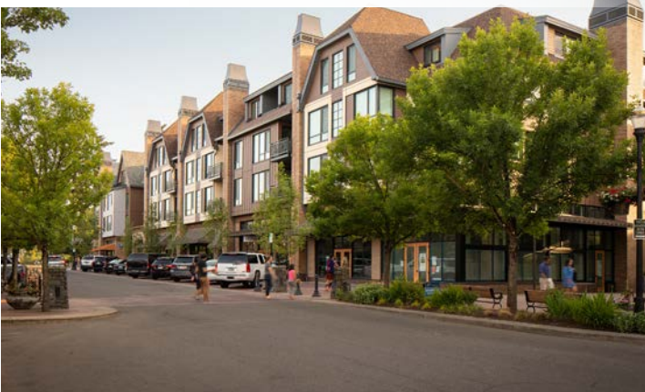
VIEW LOOKING WEST FROM FIRST STREET OF CHUCKIE PIES AND BAMBOO SUSHI & PEDESTRIAN WALKWAY
